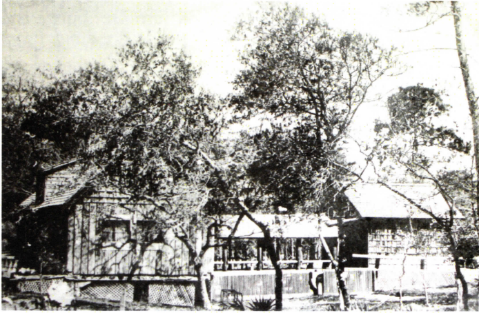
The Nathan Cobb Cottage originally included a wood outer kitchen and dog trot – photograph ca. 1900. Source Ormond Beach Historical Society.
