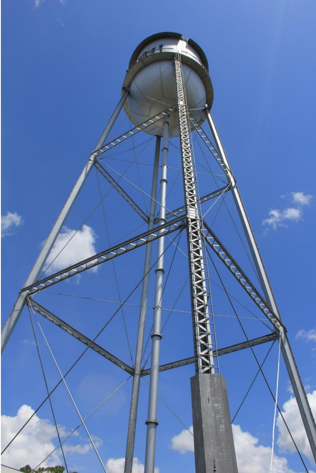
Figure 5 - Ladder on the SW steel column of the Water Tower – (photograph by author – August 2018).
