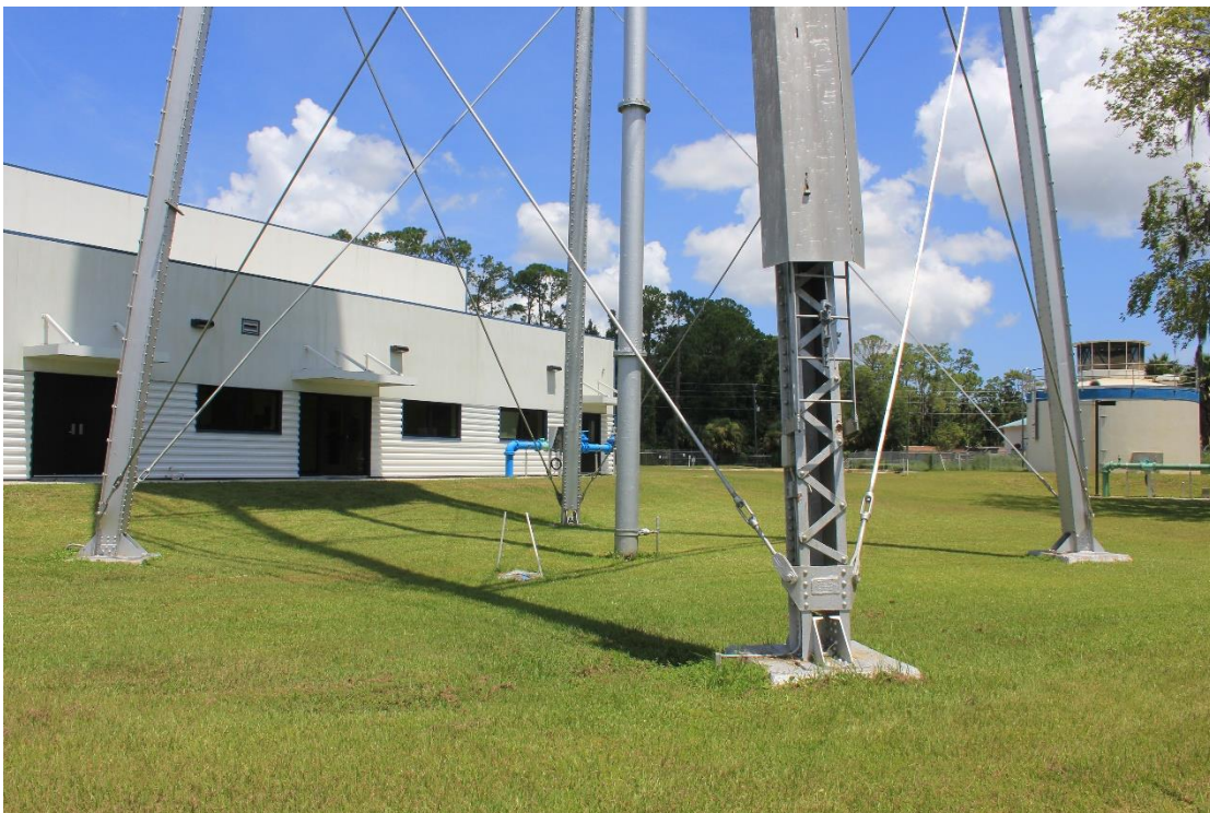
Figure 4 - Columns of Water Tower - Ground Attachments – (photograph by author – August 2018).
