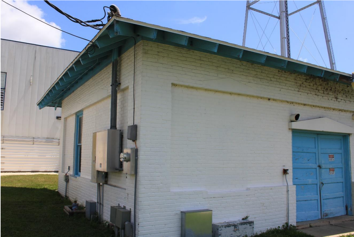
Figure 6 - SW View of Original Pumping Station – (photograph by author – August 2018).
