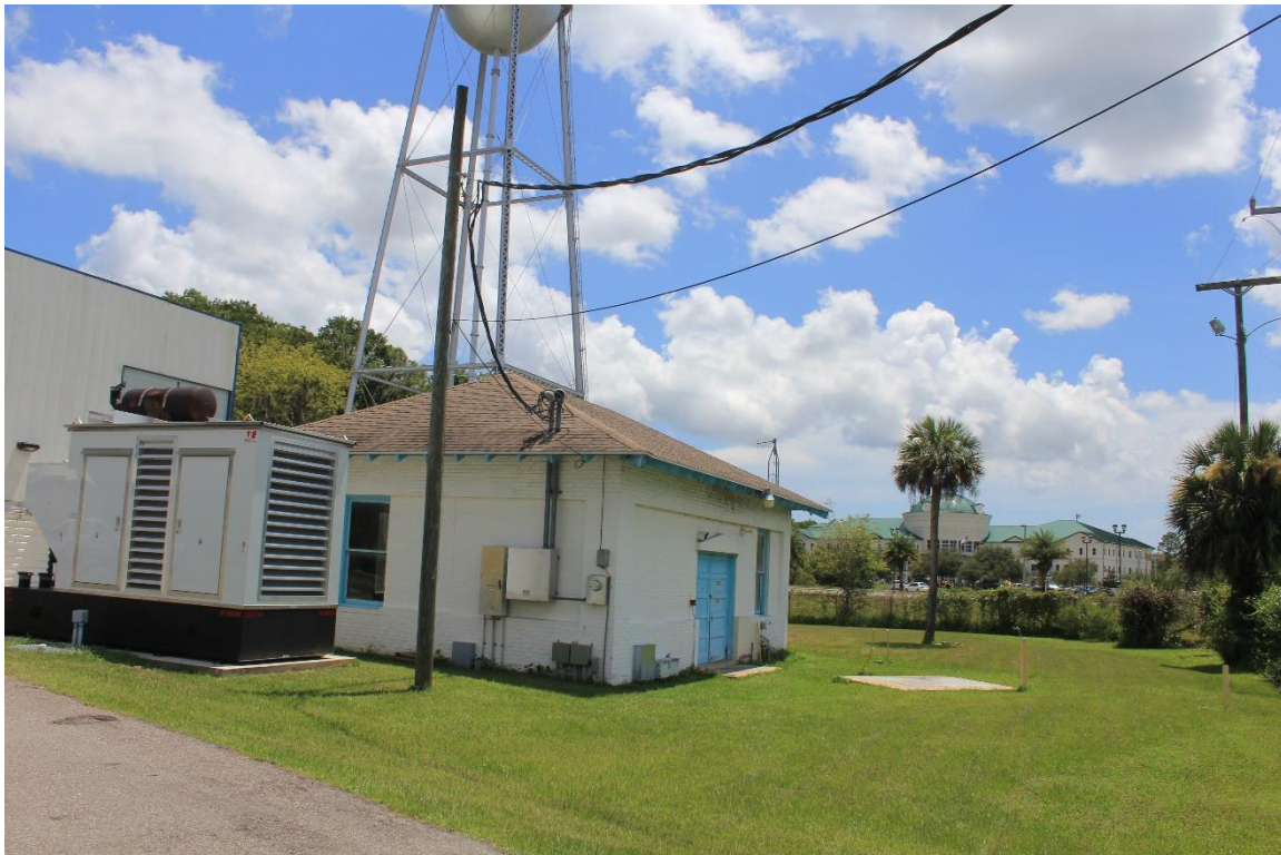
Figure 7 - NW View of Original Pumping Station – (photograph by author – August 2018).
