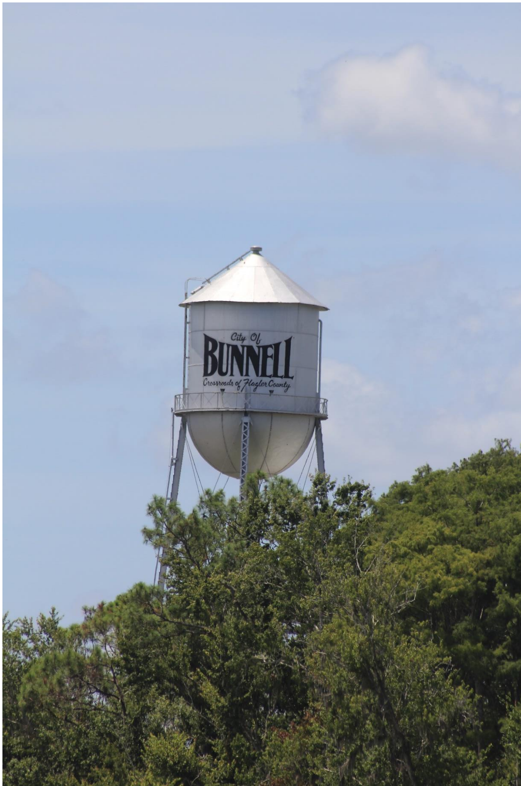
Figure 8 - East Side of Elevated Water Tank – (photograph by author – August 2018).
